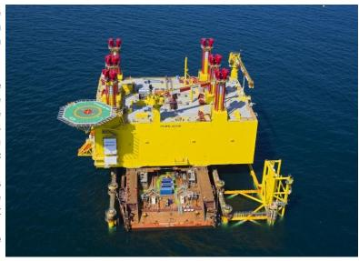
The Siemens electrical plant fitted inside the platform is capable to transmitting 864 MW into the onshore power grid making it the most powerful converter substation installed in German waters to date. **OVERDICK** on behalf of Siemens, the general contractor for the project, conducted the concept design and the structural detail engineering, as well as the transport and installation engineering.
